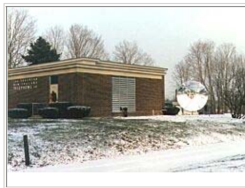
New Haven, CT Installation
